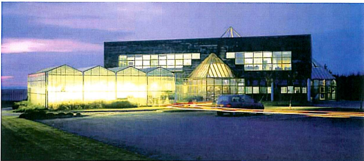
Headquarters of BBV (Bretagne Biotechnologies Vegetales - Brittany Plant Biotechnology) at Saint Pol de Léon (photo courtesy of BBV-GPO). La sede del Bbv (Bretagne Biotechnologies Vegetales) a Saint Pol de Léon (photo credit BBV-GPO).
